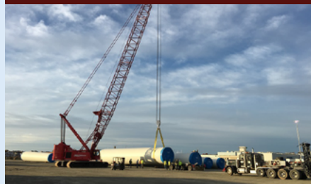
10/28/15: Tower pieces are packed for delivery.
