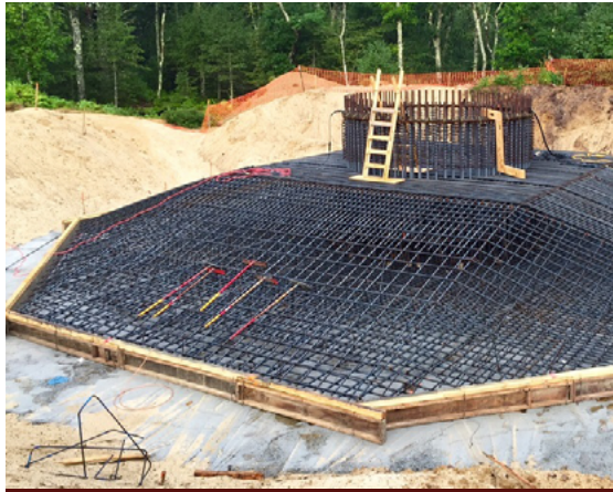
8/12/15: Steel framework is laid for the turbines' foundations.
