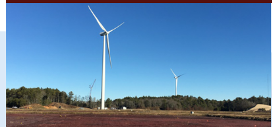
12/15/15: Two of the four turbines are up.
