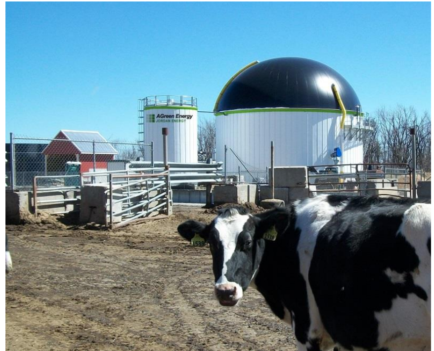
Anaerobic digester, Rutland, MA
